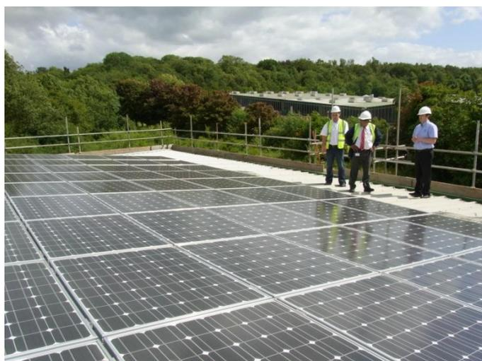
The groups were then taken onto the roof to look at the panels. The system has been thoroughly tested to ensure that it can withstand wind loading. The panels are fixed on the supports rather than on the actual roof and calculations have been made to ensure that the weight of the system can always be supported.
