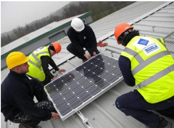
The installation was surprisingly uncomplicated and included minor alterations to the structure of the roof, fitting of the mounting system, electrical work and commissioning. The installation is robust and will easily substantiate a 25 year plus investment. It consists of 54 solar panels and is capable of generating 8000kWh it's believed to be the first of its kind in Telford.
